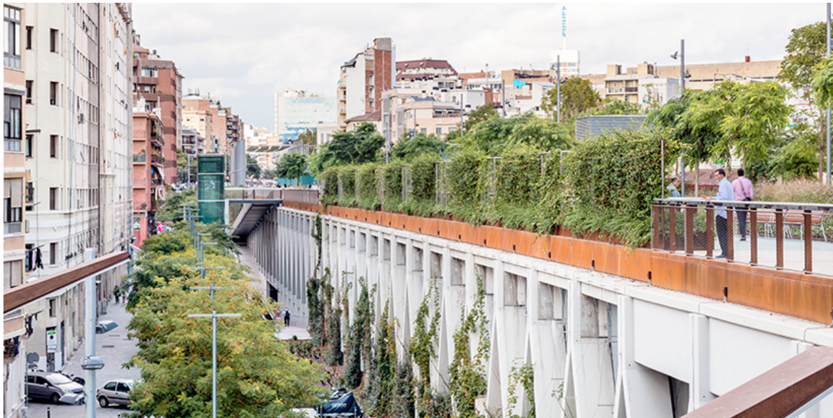
Figure 2: Image of the elevated Rambla de Sants by Adria Goula.
