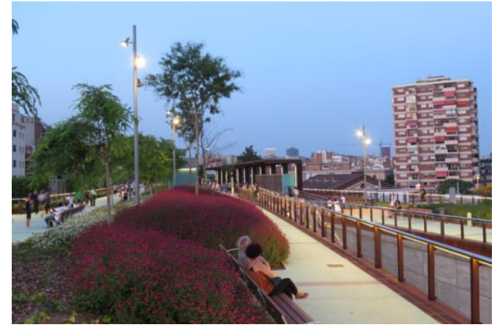
Sants railway encasement
