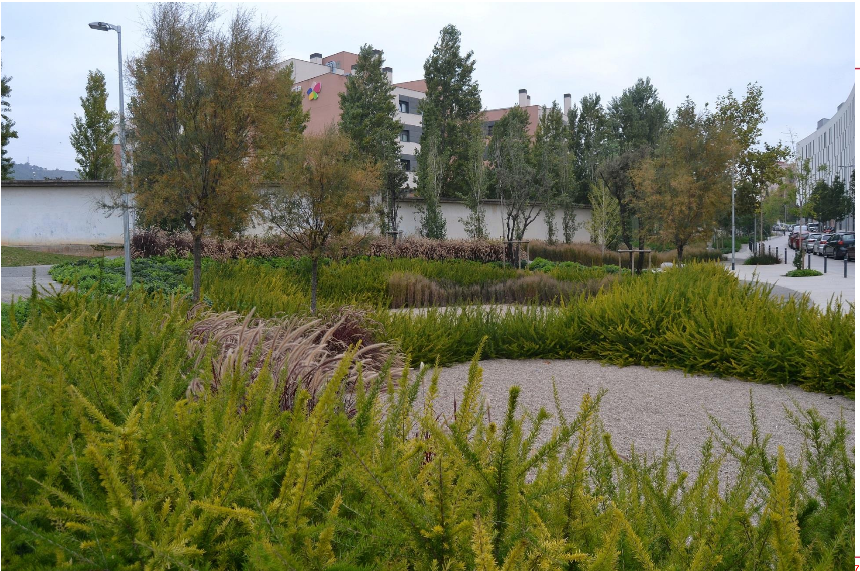
SUDS (Sustainable Urban Drainage System) in Av. Can Marçet
